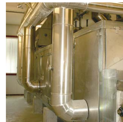
Belt drier with hot gas heating in stainless steel
