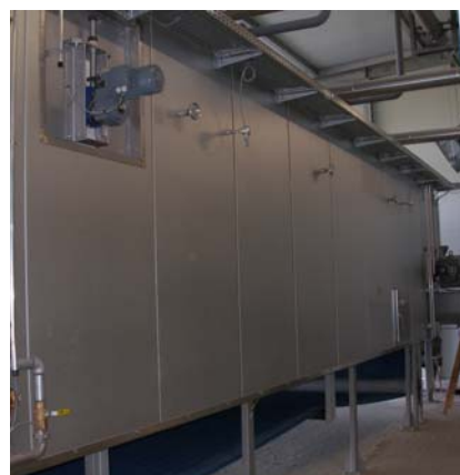
SBT 60/5 new insulation
